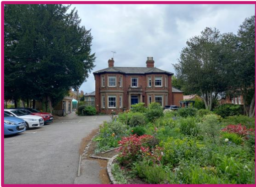
The front of the main building with carpark
